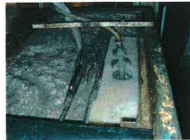
Example of installation of floating oils collection nozzle
